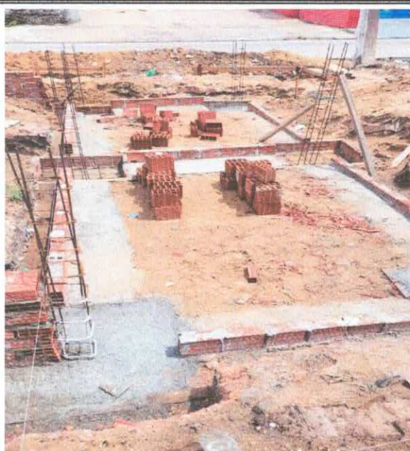
Foto 11: 6.2.0.5. Concreto fck = 30mpa, preparo com betoneira. (01/01/24 a 10/02/24)
